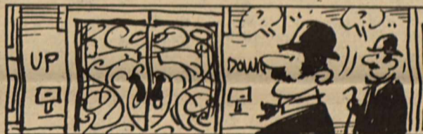
The first successful electric elevator was installed in the Demarest Building in New York City, in 1889.
