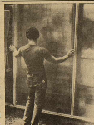
Installing double-skinned acrylic sheets can be a do-it-yourselfer's delight.
