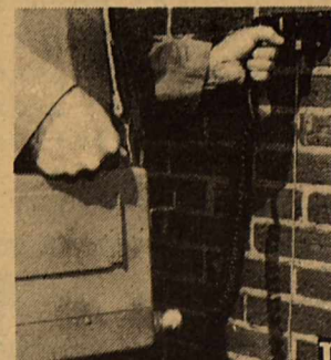
An outdoor receptacle lets the meter reader electronically read a meter anytime without entering your home.
