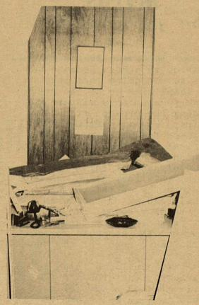
AND THE WALLS CAME TUMBLING DOWN!! Well, almost everything else came tumbling down but the walls in the Kinney County Judge's office this past week. The total ceiling in the office collapsed! Including the light fixtures, ceiling tile, support structures, and air conditioning ducts.
