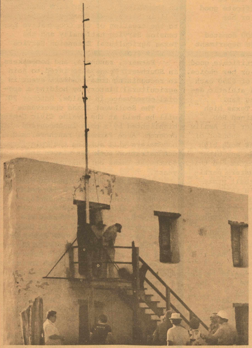
ERECTING A PORTABLE/EMERGENCY ANTENNA ON "THE ALAMO" AT ALAMO VILLAGE.
