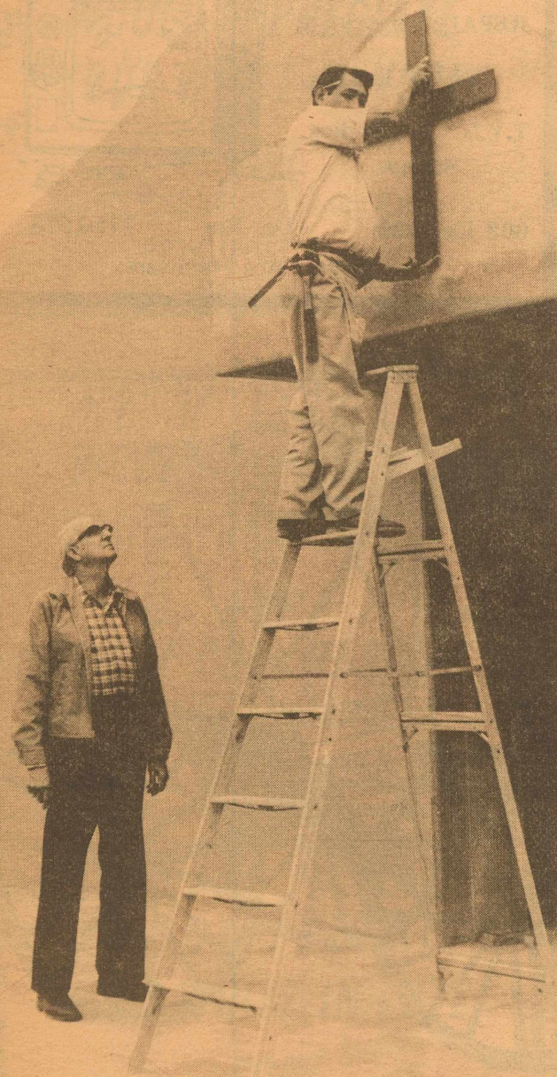
PASTOR JOE TOWNSEND looks on as the cross is installed on the new Frontier Baptist Church. Dedication ceremonies are scheduled for Sunday.
