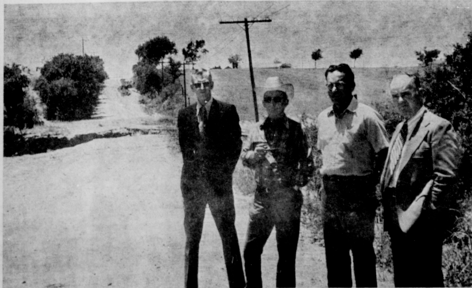
EXAMINING DAMAGE —From left to right are pictured, Frank Cox of the Texas Dept. of Public Safety, V. C. (Zipp) Durrett, Lakeview Precinct Commissioner, Memphis Mayor Kenneth Dale and Jesse R. Ward, Manager of the Civil Defense and Disaster Relief Dept. of Austin, as they examine flood damage caused by a six-inch rain last Friday night. In the background is the deep washout on Mendon Street which left a 30-ft. deep canyon.
