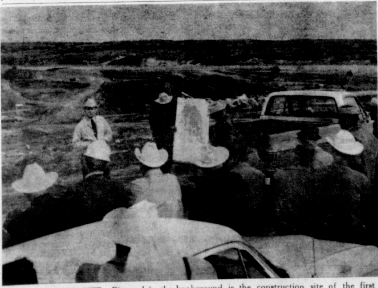
CONSTRUCTION SITE —Pictured in the background is the construction site of the first dam to be built in the Lakeview Watershed. As Area Conservationist Douglas Cunningham explains the Watershed, District Conservationist Henry Gregory and Paul Montgomery hold a map showing all the 25 planned dams and the channel improvements. Approximately 75 persons were on hand for the ground breaking ceremonies Wednesday.
