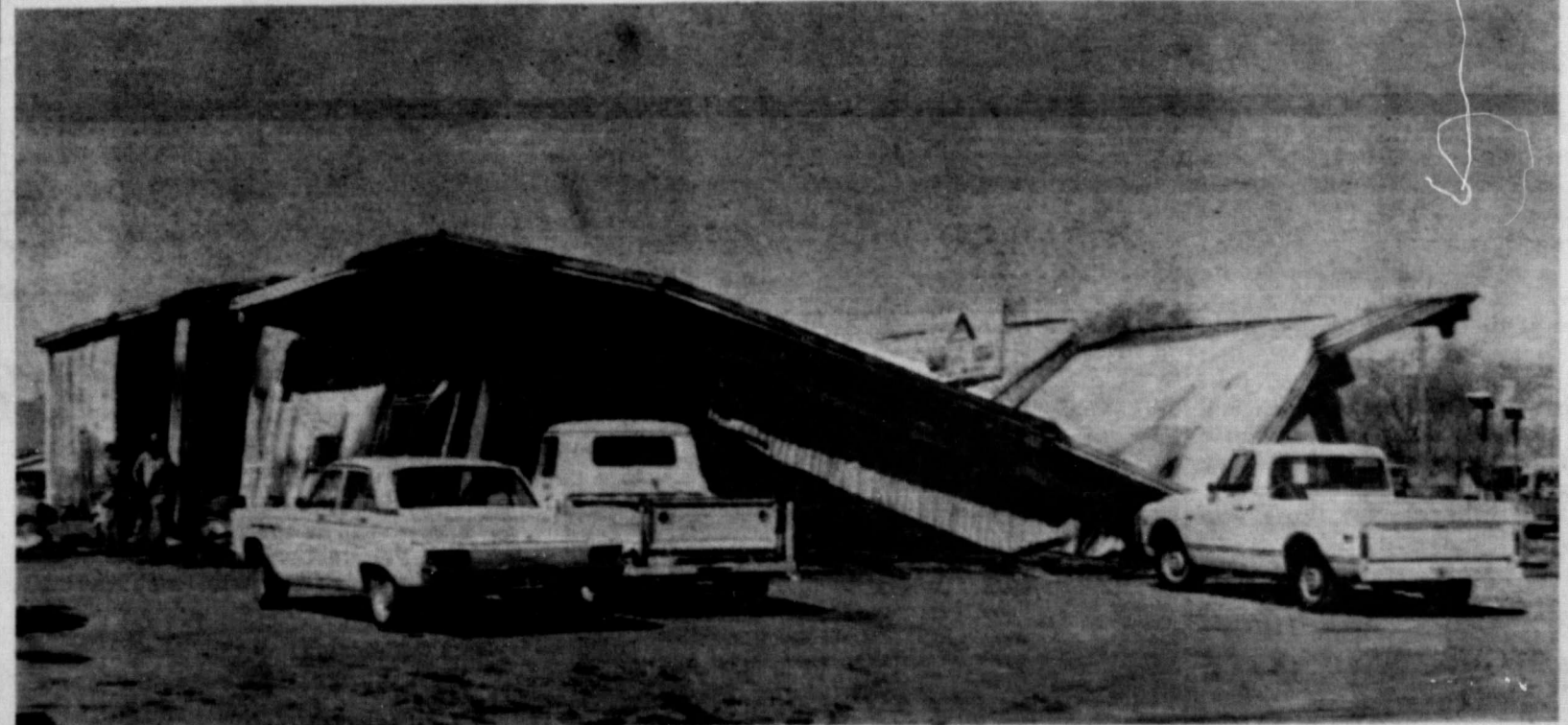
DESTRUCTIVE FIRE —A truck on U. S. 287 passing through Memphis detected a fire at Shields Implement Co. shortly before 5:30 Tuesday morning. Firemen were summoned but by the time they arrived on the scene the entire inside of the steel building was ablaze. At about 5:45 a. m. the front windows in the building blew out, fortunately no one was injured by flying glass. Firemen battled until 7:30 a. m. when the fire was finally extinguished. As the above picture shows, the building and its contents were destroyed. Also in the building were two tractors and a pickup being repaired. The new Allis Chalmers equipment had been moved by firemen and was not lost, it was reported. This is the heaviest commercial property fire in Memphis since the 1954 fire which destroyed a portion of the downtown area.
