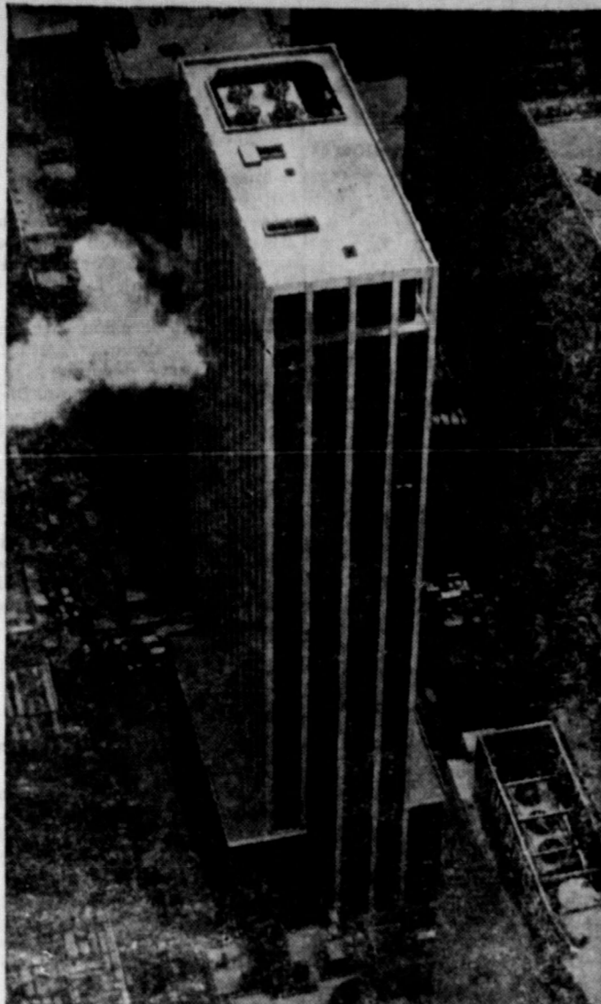
NEW BUILDING —Viewed from the sky above is the new 45-story J. C. Penney Building in New York, which was dedicated Jan. 27. The company's new central office, unique as a building specially designed to serve a retail chain, provides a more efficient base from which to speed merchandise to nearly 1,700 stores of which the store in Memphis is one.
