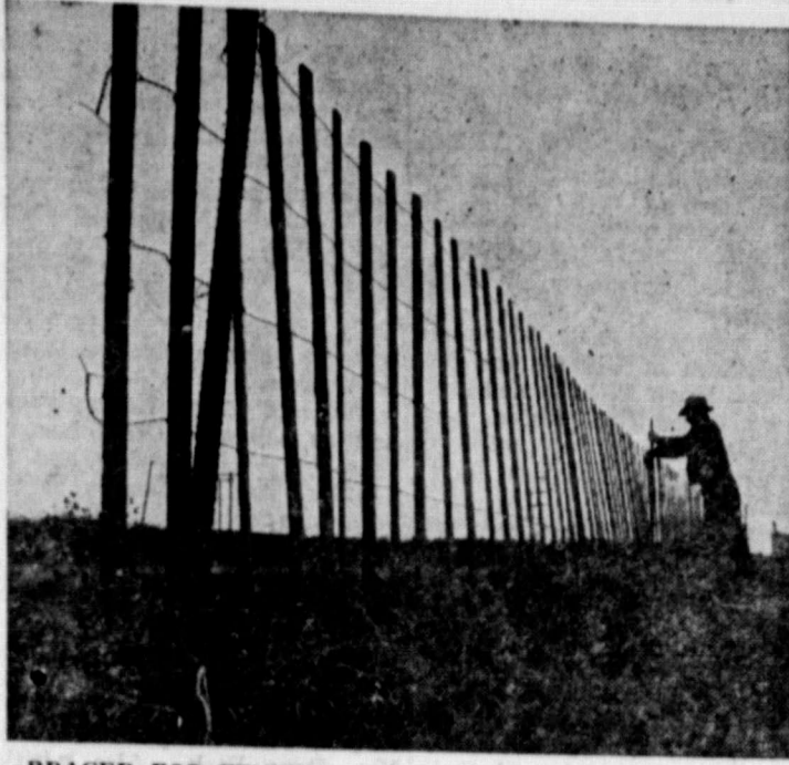
BRACED FOR WINTER . . . Kansas State Highway Department employe checks over a newly-installed snow fence on the Earl Hepworth farm near Dover.
