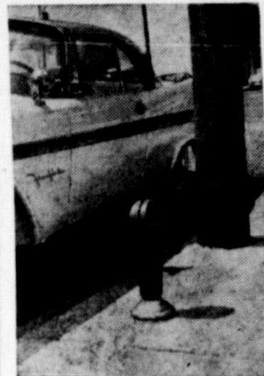
LOWDOWN TRICK? . . . Parking meter sunk to the depths at Memphis, Tenn., where it was improperly anchored in cement over soft earth.
