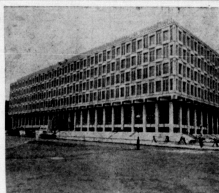
NEW AMERICAN EMBASSY . . . Nearly completed in London is the new American embassy designed by Eero Saarinen in Portland stone with aluminum trim. It has incensed some traditionalists.
