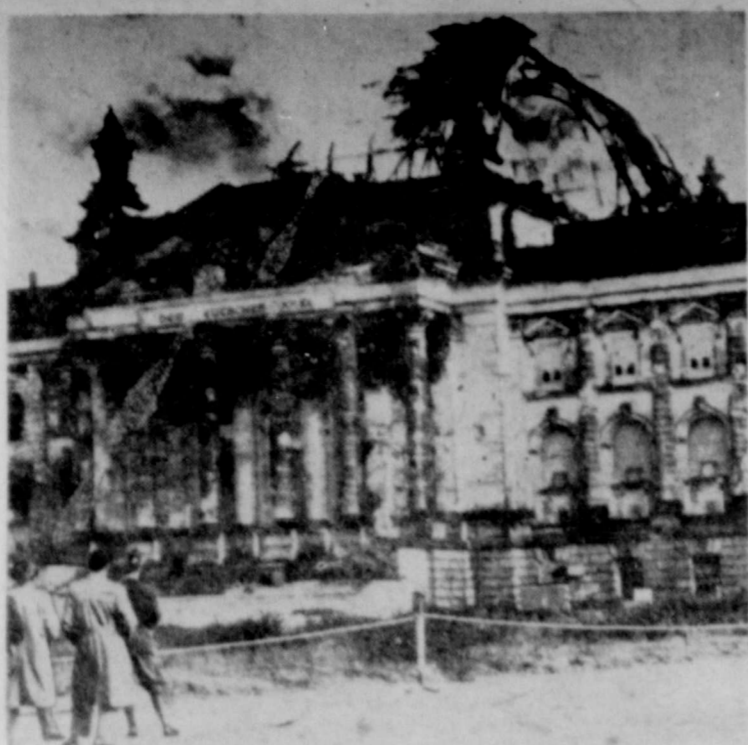
INDOMITABLE DOME . . . Berlin demolition engineers using thermite fail to topple dome of Reichstag which survived 1934 Nazi fire and World War II bombings.
