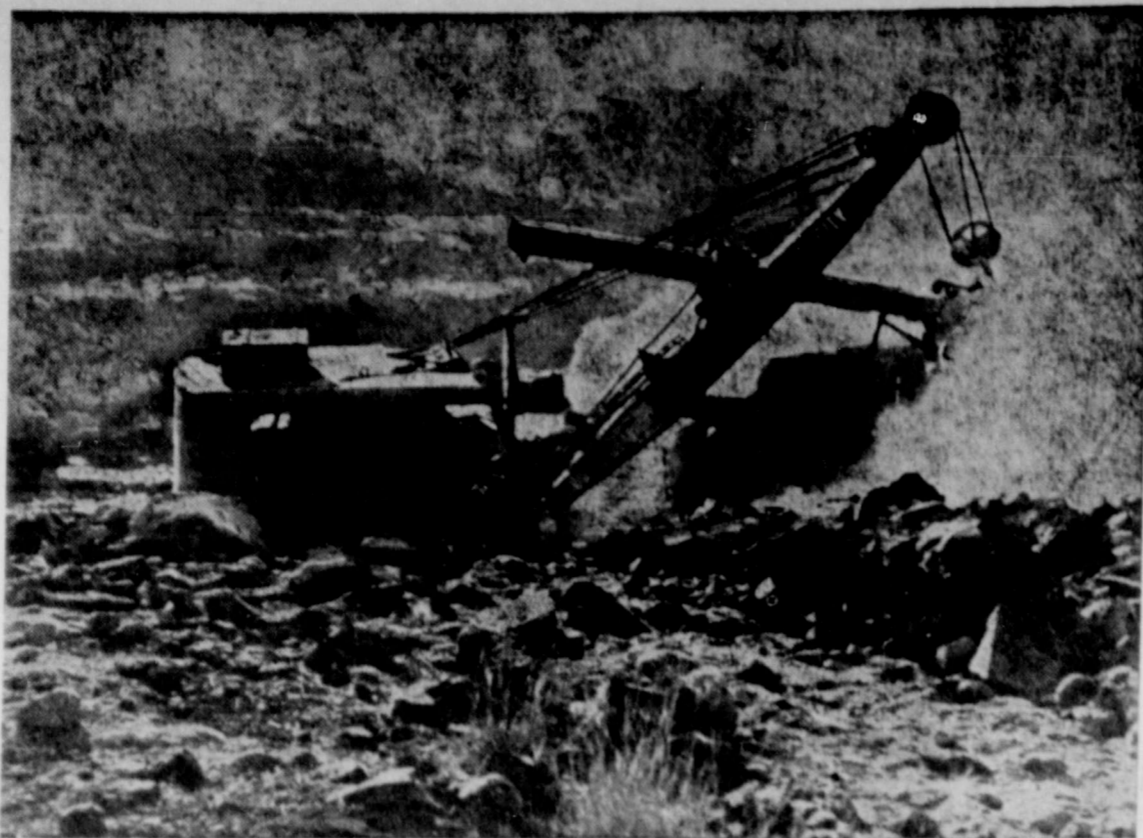
ISRAEL DIVERTS JORDAN . . . Power shovel in Hulch region of Israel digs new river bed to divert Jordan River water, project which UN ordered halted after Arab protest.
