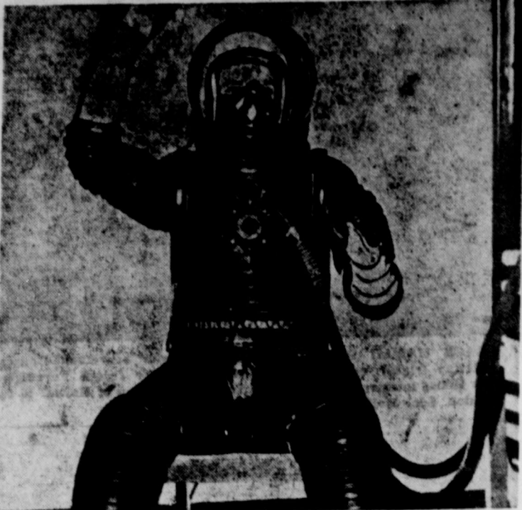
MAN FROM MARS? . . . Developed by the U. S. navy for high-flying rocket or jet aircraft pilots, this new pressure suit protects pilot at 100,000 feet and despite its bulk is very flexible.
