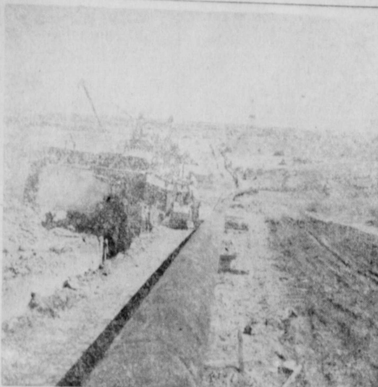
BIG DITCHER —Moves into Doyle field in south Central Oklahoma as work progresses on Lone Star Gas Company's new 70-mile, 20-inch transmission line which will strengthen 25 million cubic feet of gas daily from Skelly Oil Company's Velma (Oklahoma) gasoline plant. New line is already carrying
