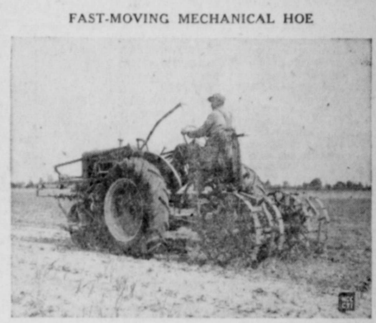
Because he always thought there was an easier way to chop cotton than by hand with a hoe, Riley Dabbs, Monroe County, Miss., farmer and sawmill operator, began work four years ago on this mechanical cotton chopper. Getting its first test on Cotton Belt farms this season, the chopper reputedly can thin 30 acres of young cotton at a cost of $7 for the day's operations.
