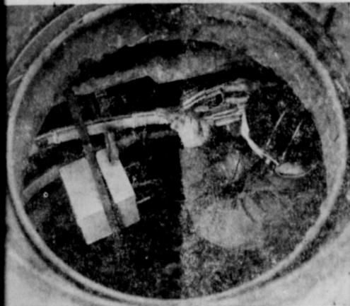
The average man on the street has no use for a "bliffy sniffer." However, this repairman under the street uses a "bliffy sniffer" in his right hand to match, in less than a minute, any particular pair of the hundreds of strands of the cable he is working on.
