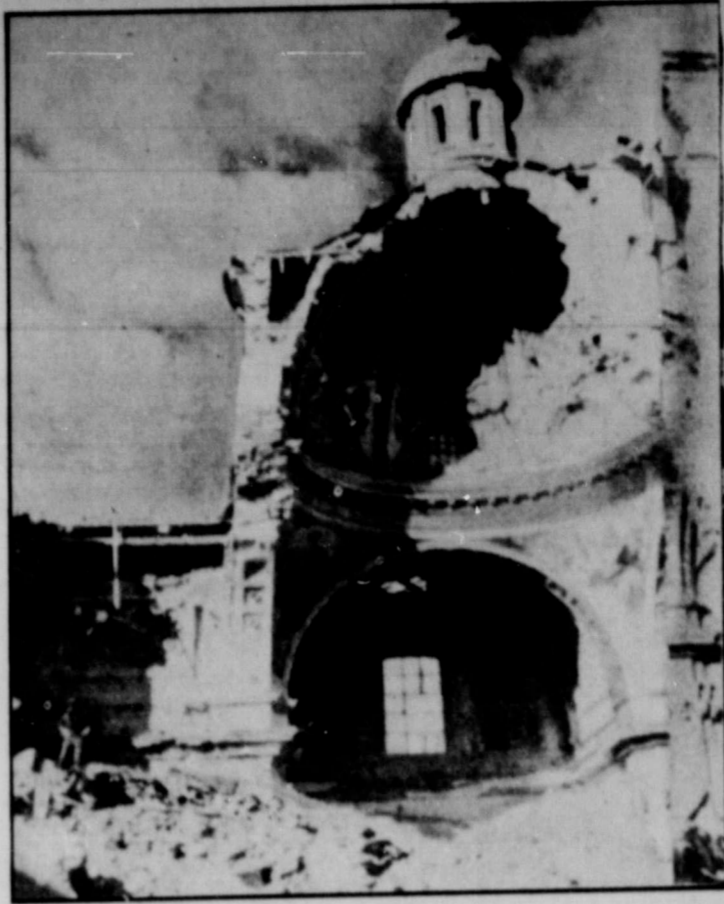
This shows a job done by the fleeing Germans on the 1100-year-old St. Thomas Cathedral in Ortona, Italy, after the Canadians entered the town. Destruction of the church was one of the enemy's last acts, an attempt to impede the advancing Allies. (OWI radiophoto.)
