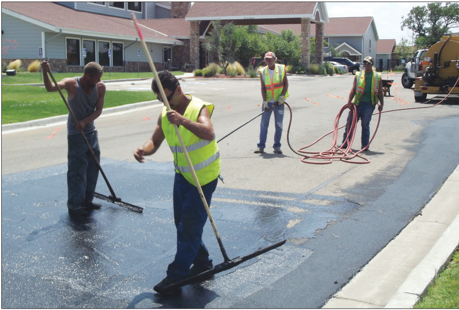
A crew of workers (left to right) Robert Godwin, Ernesto Gallegos, Bill Hite and Daniel Harper spread hot tar on the driveway of the AmericInn.
