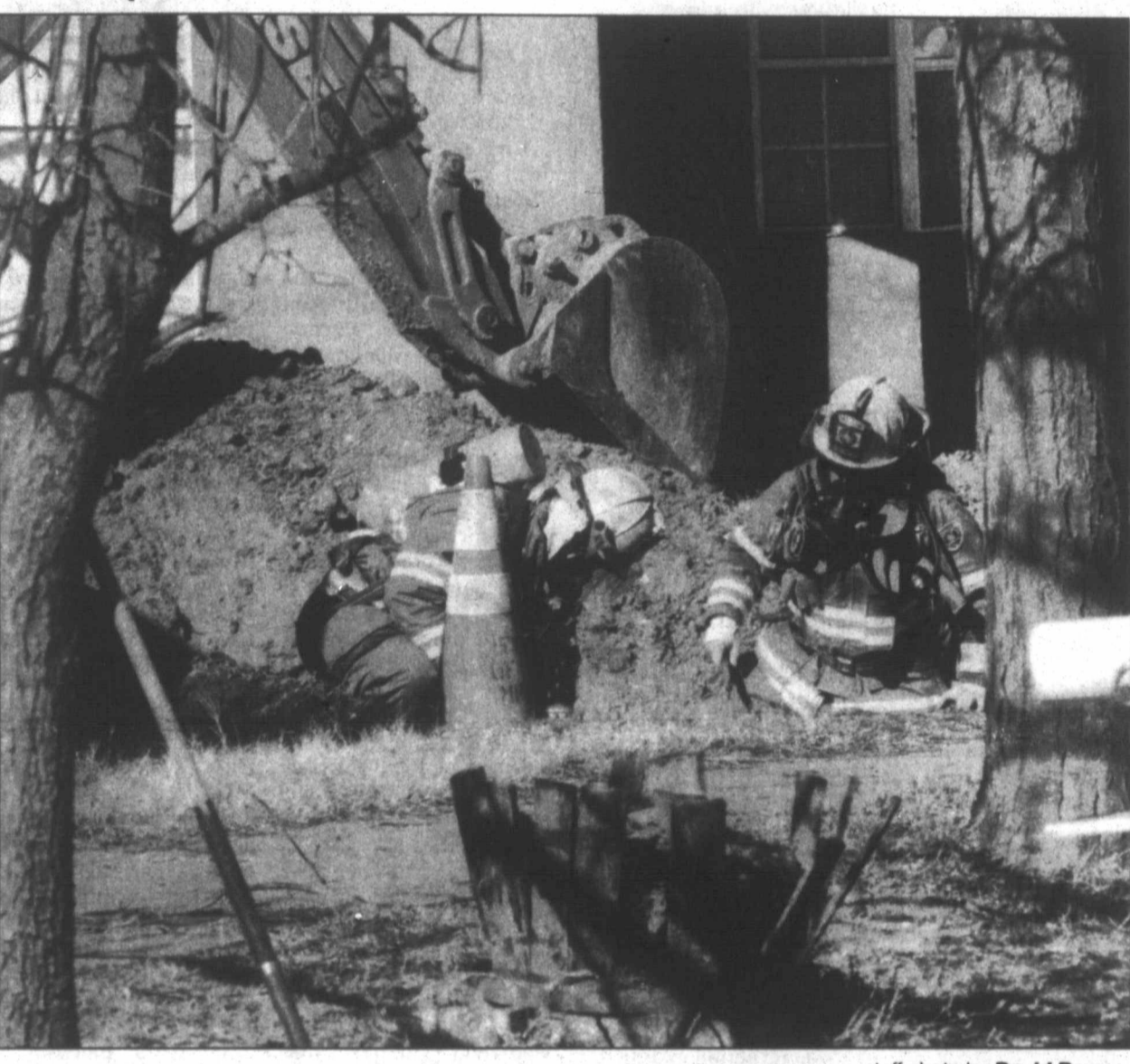
Pampa firefighters Tim Roberts and Josh Taylor work to stop a gas leak in the 400 block of Starkweather. City water crews were repairing a water line when they hit a gas line with a backhoe about noon Wednesday. staff photo by David Bowser
