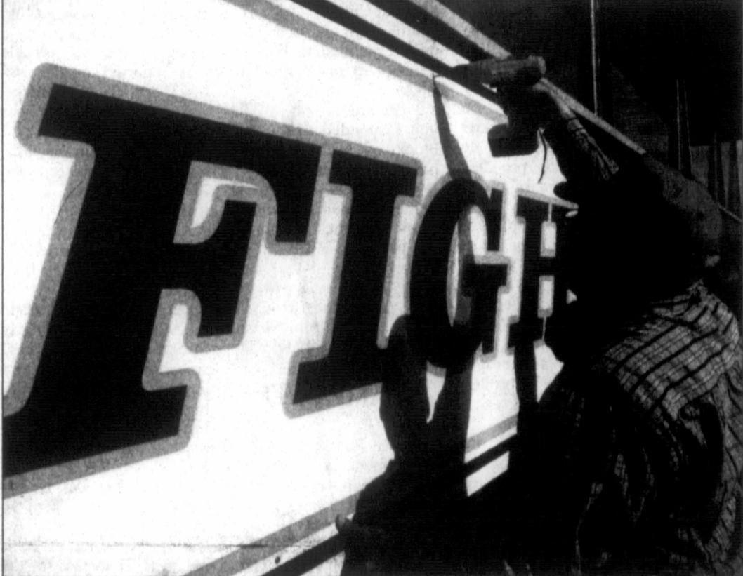
Don Stone puts up a section of a new sign on the front of the press box at Harvester Stadium this week as new artificial turf is put in place to get ready for the fall's football season.
