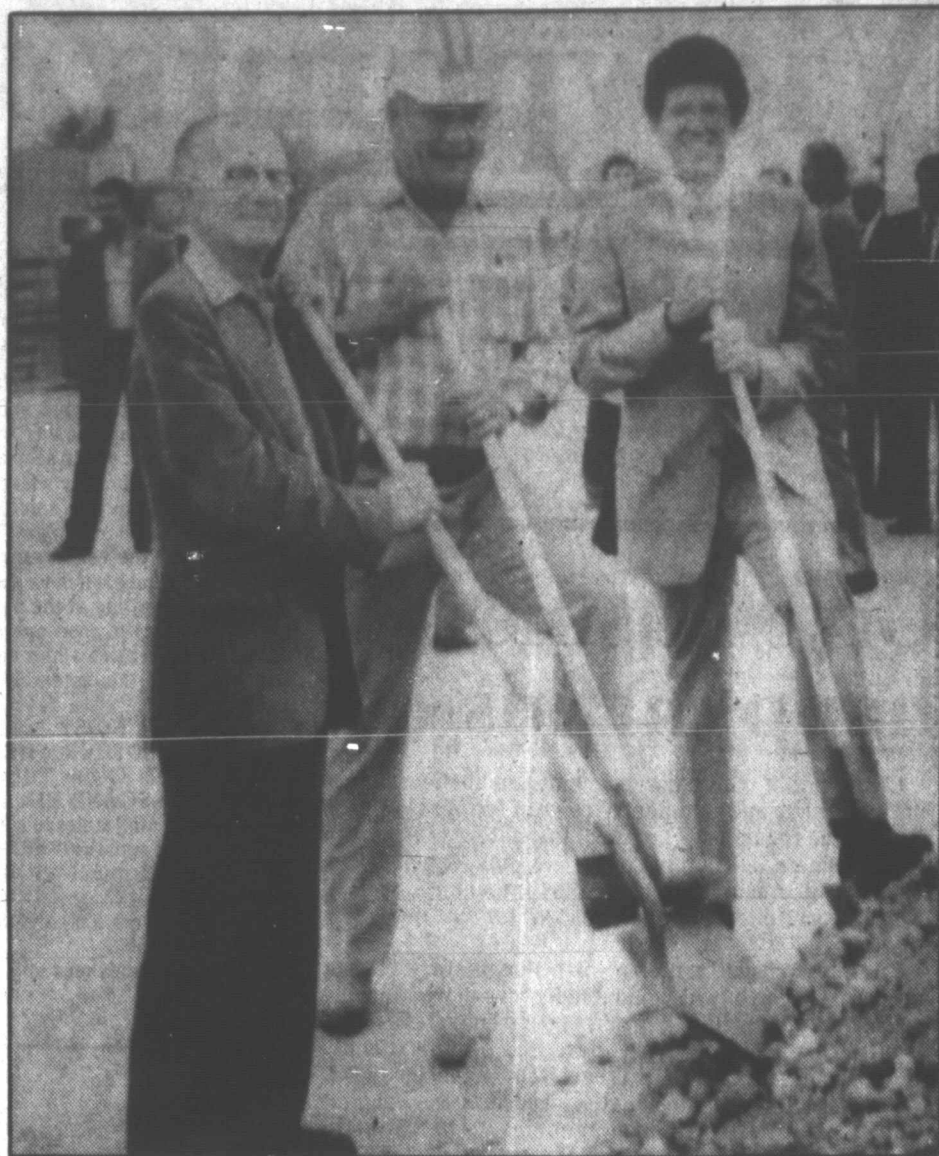
Breaking ground for a new Perryton National Bank building are PNB President Ed Garland, left, construction foreman Dan Ritter and architect Chick Lee. The new home for PNB will cost $1.5 million and is expected to be finished by the end of December. (Correspondent Photo by Sherill McLearen)
