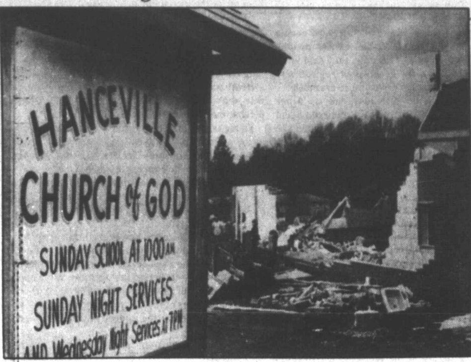
This is a view of tornado damage to the Church of God in Hanceville, Ala., Tuesday. Damage to the church was estimated at $30,000. Buildings in a nearby shopping center were also damaged. (AP Laserphoto)
