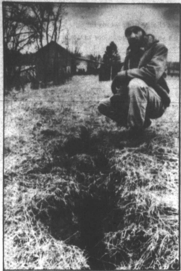
Mark Spezza kneels next to a crack in the hill behind his Wilkesville, Ohio barn. Spezza believes the crack was caused by longwall mining of coal beneath his 57-acre tract. The cracks in the land run through his century old barn, in background, causing the floor to crack open six inches. (AP Laserphoto)
