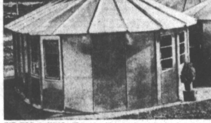
FIT FOR A KING—This portable aluminum "palace" is being exported by a London, England, firm for use as a hunting lodge by King Saud, of Saudi Arabia. Each of the two prefabricated buildings can be erected or dismantled within an hour and transported by camel.
