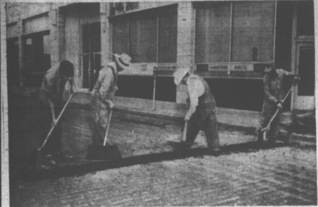
FIRST AID FOR Pampa streets that buckled under intense heat yesterday afternoon were being temporarily repaired today by the street department. The worst places were started and finished between 4 and 5:30 p.m., yesterday. Shows above repairing the N. Russell and W. Kingsmill intersection are, left to right, Bill Webb, O. Z. Kunkel, G. C. Murphy, and H. C. Dawson, of the Street Department. Nine spots on Pampa streets started buckling at 4 p.m. yesterday and rose as high as eight inches. Concrete slabs will be laid at a later date, city officials said this morning when permanent repair work gets underway. (News Photo)
