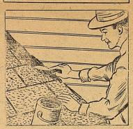
House and barn repair time is at hand. Work done now will eliminate troubles this water. It might be a good idea to check joints between siding and roofs on all farm buildings, including the farm home. Cracks should be sealed with paste roofing compound before fall painting. See to it now.
