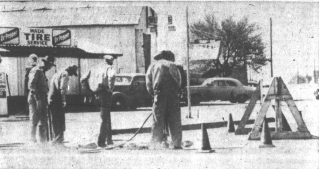
INSTALLATION WORK was begun today on the new traffic signal light at the intersection of West Foster and North Hobart. Preparatory work should take about four days, according to Fred Brook, acting director of Public Works. (News Photo)
