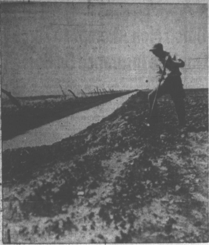
DIGGING BY THE TRENCH which carries irrigation water to T. D. Hodges' parched soil is his son, Roy B. Hodges. Bent siphon-pipes are extended from the trench over the top into each furrow (where Roy is standing). His irrigation pump is one of the first in this area. (News Photo)
