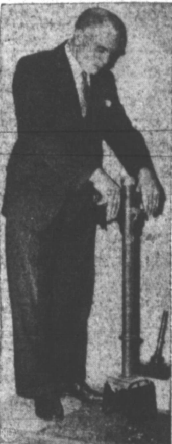
SQUARE HOLE DIGGER —If you have to dig square holes, then the thing you need is a "square hole digger," an ingenious invention recently displayed at a London inventors exhibition. The new invention, used mainly when fencing land, can cut holes four-and-a-half to 18 inches square.
