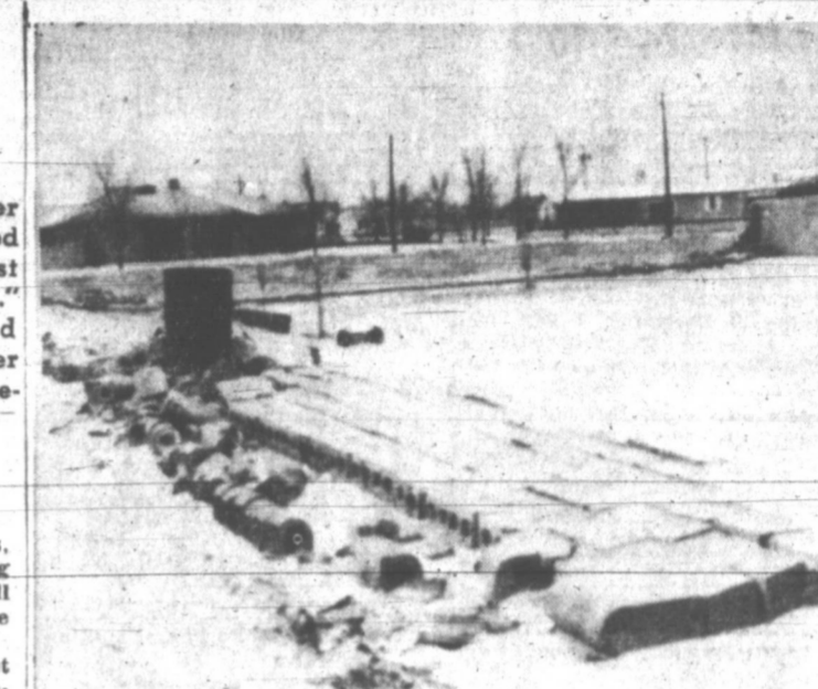
WIND DAMAGE — Two sides of a concrete block fence (foreground and background) to the rear of the residence of Ed Cleveland, 1812 Christine, were knocked down early Monday night by a small twister, one from the north, the other from the south. As seen by Mrs. T. J. Worrell, 1707 Christine, there was "a lot of noise" as the clouds came together over Cleveland's fence (seen in the rear) and then snapped down the fence (in the foreground). (News Photo)
