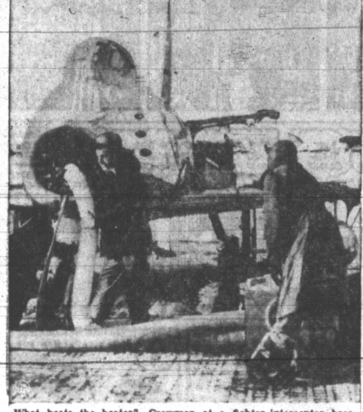
What heats the heater? Crewmen at a fighter-interceptor base warm an F-86 Sabrejet with 300-degree air on a bitter-cold morning.
