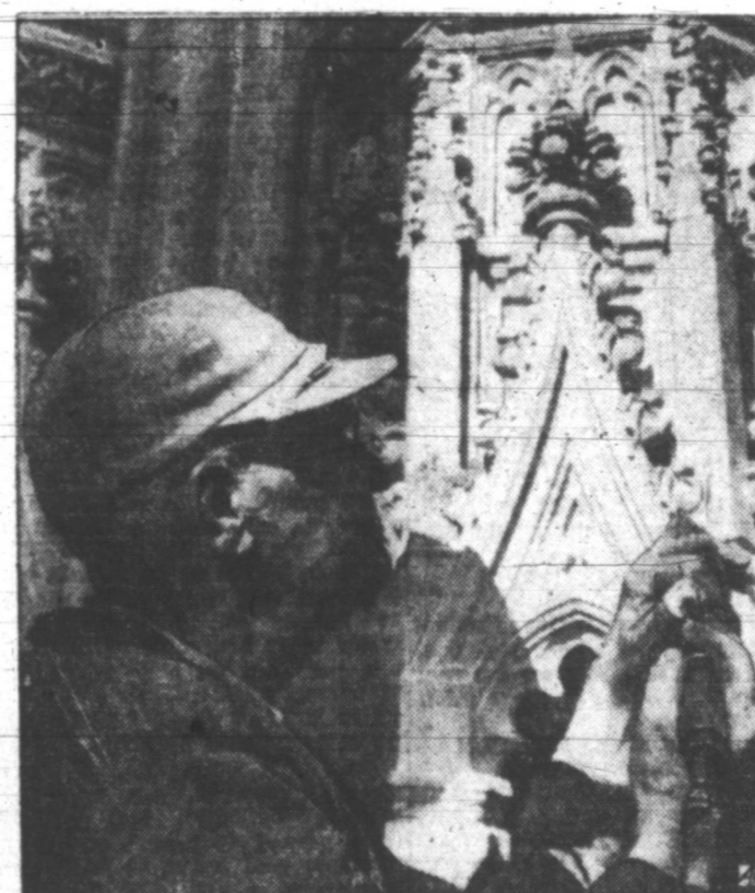
ENDURING PIECE OF WORK —Joseph Ratti, ornamental stonecutter, puts finishing touches to decoration on one of great arches of the National Cathedral in Washington.
