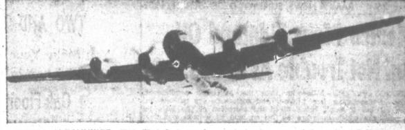
AERIAL HITCHHIKER-With "baby" fastened securely in place, a specially modified B-29 takes to the air at Seattle, Wash., prepared to launch the tiny Douglas Skyrocket at a high altitude. Once dropped from the mother ship, the pilot of the small plane ignites his rockets, and is on his own. In tests, the small ship has attained a speed of 1238 miles per hour and altitude of 79,494 feet.
