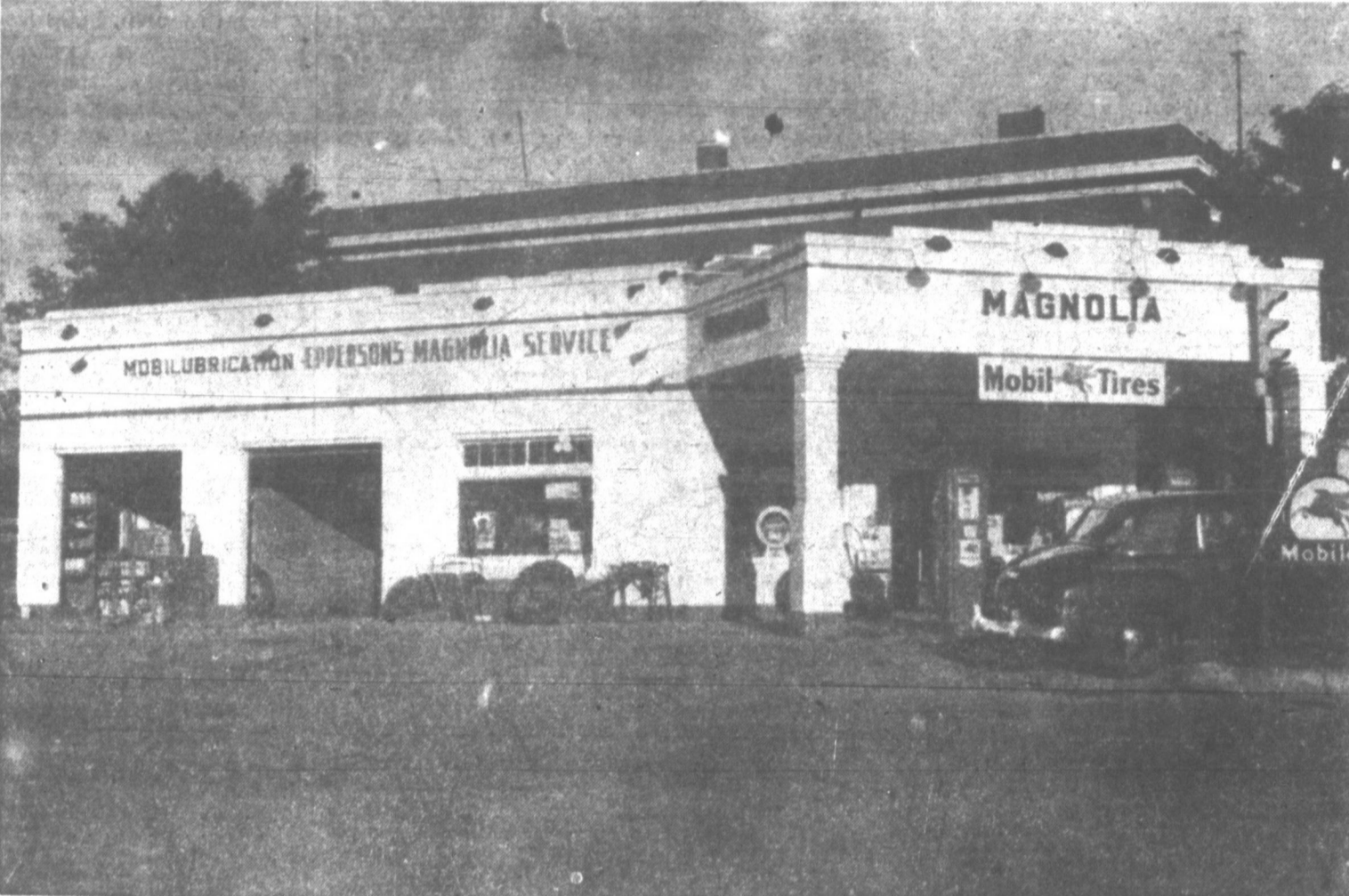
AUTOMOBILE NEEDS QUICKLY FILLED AT EPPERSON'S — There is one station located in Pampa that features quick and dependable service. That service station is the Epperson's Magnolia Service Station, located at 120 S. Cuyler. Across the street is a free parking lot in which they will park your car for you while you attend to business or shopping needs. It is nice to know that when
