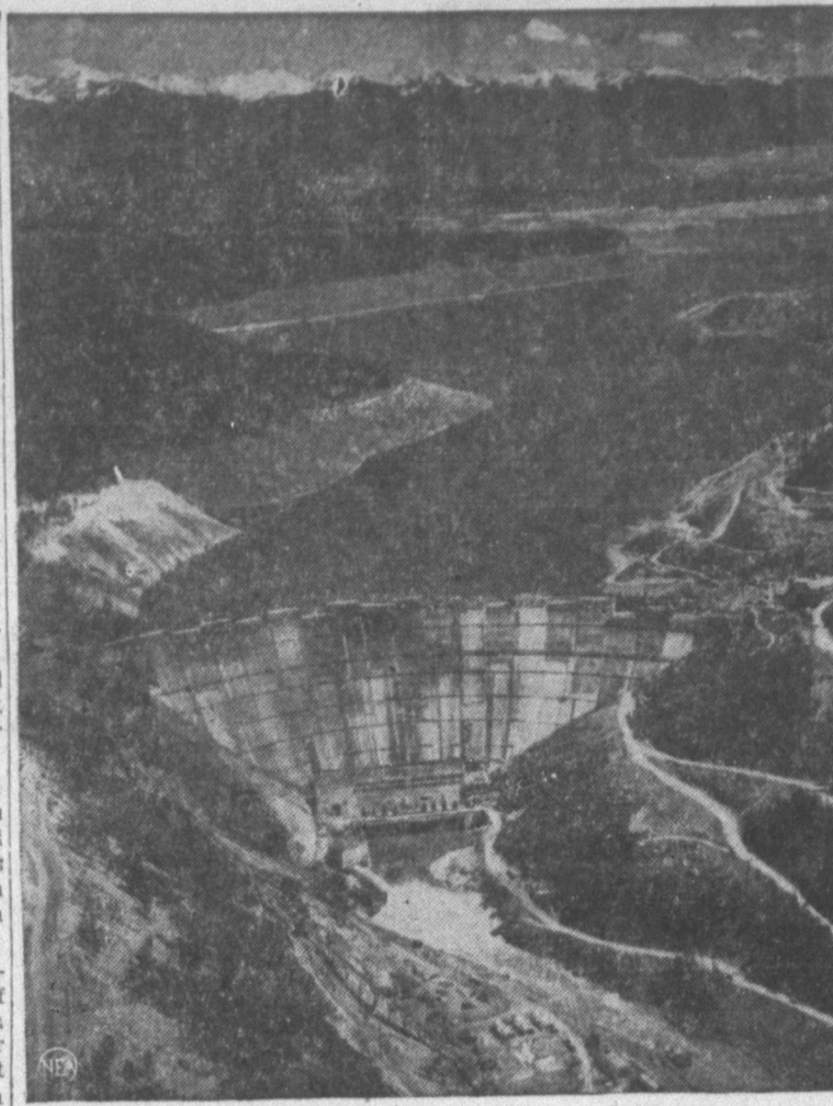
BEAUTIFUL DAM SITE —Scenic beauty surrounds Montana's newest lake—a man-made body of water slowly rising behind newly finished Hungry Horse dam in the northwestern part of the state. This aerial view shows the dam and the reservoir behind it. When filled the reservoir will extend 34 miles up the south fork of the Flathead River. It will be approximately 500 feet deep at the dam, up to three and a half miles wide and will store about 3,500,000 acre-feet of water.
