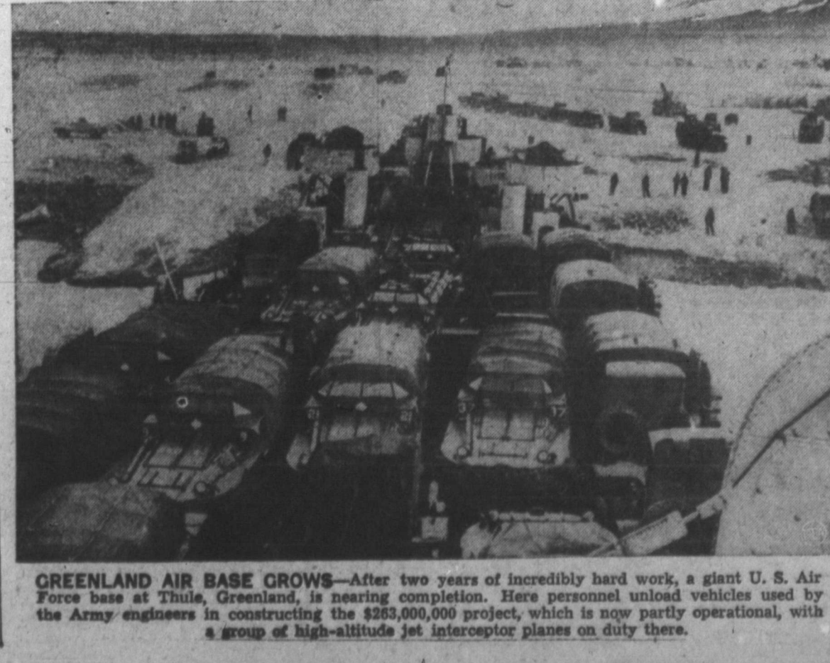
GREENLAND AIR BASE GROWS—After two years of incredibly hard work, a giant U. S. Air Force base at Thule, Greenland, is nearing completion. Here personnel unload vehicles used by the Army engineers in constructing the $263,000,000 project, which is now partly operational, with a group of high-altitude jet interceptor planes on duty there.
