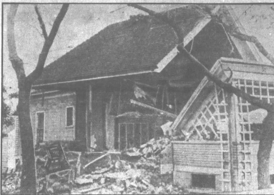
Typical of the ruin wrought by the quake which caused more than $2,000,000 damage and claimed two lives in Helena, Mont., is that shown at this home, where the occupants narrowly escaped with their lives when the structure collapsed. More than 400 buildings were damaged in the Montana capital, a city of 14,000, and the Red Cross has taken over the relief of scores of families. Hundreds of Helena residents fled in terror into the open country as shock followed shock.
