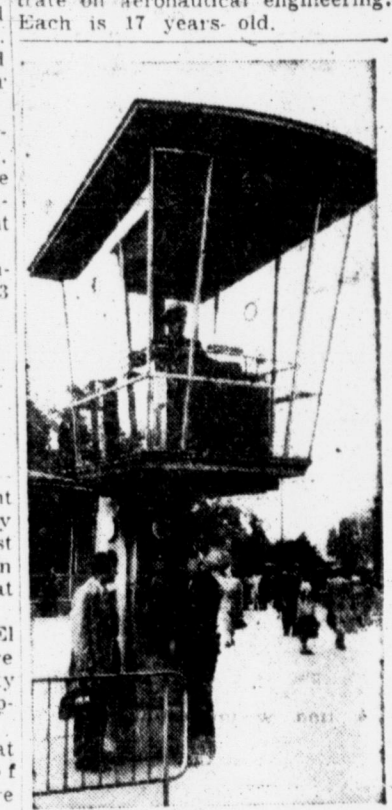
TRAFFIC EXECUTIVE — High above the traffic, this policeman in Hanover, Germany, sits in air-cooled comfort (note electric fan), and directs several auto and pedestrian crossings by remote control. A loud speaker enables him to direct down offenders in traditional fashion.
