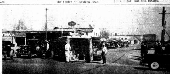
LITTLE CRACKUP-When a Pampa Motor Freight Lines heavy trailer truck started to round the corner at Cuyler and Atchison, going east, a faulty coupling apparently gave way—causing the enclosed trailer body to overturn. No. one was hurt, but traffic got thick at times. Merchandise that can be seen is a shipment of bathroom commodes.
