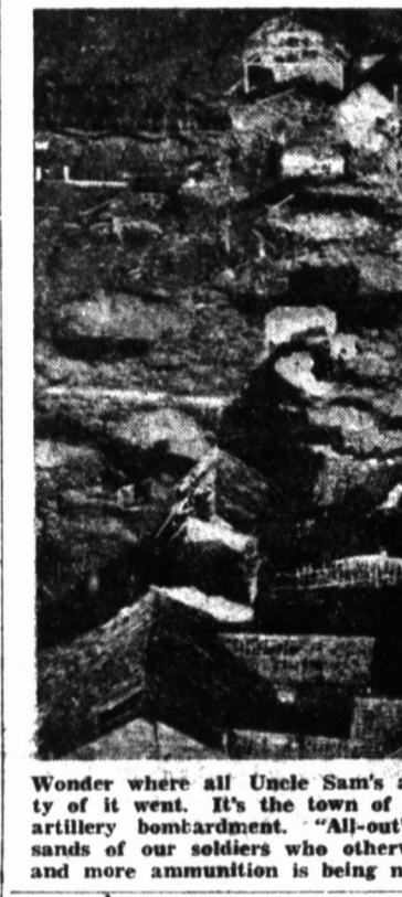
Wonder where all Uncle Sam's ammunition goes? Well, the photo above shows one place where plenty of it went. It's the town of Durn, Germany, photographed after Allied "saturation" aerial and artillery bombardment. "All-out" blasting of German strongpoints like this saves the lives of thousands of our soldiers who otherwise would have to storm prepared positions in frontal attack. More and more ammunition is being needed as the fighting grows fiercer.
