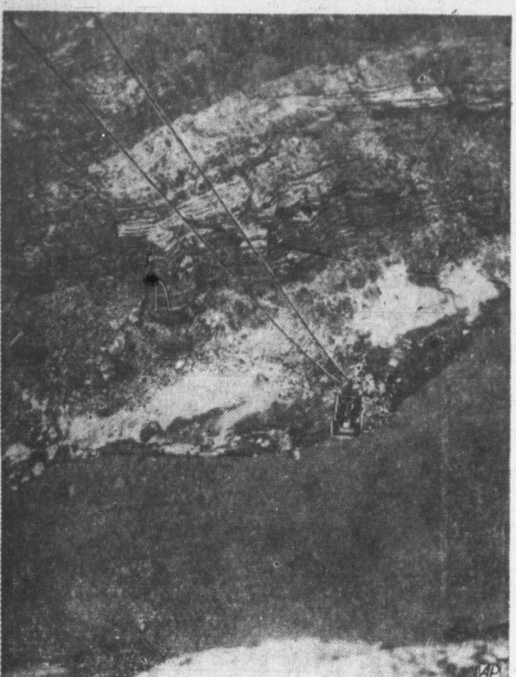
A STRONG HEART NEEDED —A metal "skin" lowers engineers 716 feet to the Colorado River at Marble Canyon, Ariz., to take soundings for a possible hydroelectric dam.
