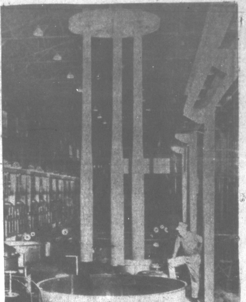
HEAT TREATING GUN TUBES — T catch of three rifle tubes are lowered into treating pits at Cabot Ordnance plant for the final step in production of gun tubes. These will be heated, air-cooled, re-heated, water-cooled and again re-heated and water-cooled before they are tempered properly. (Smith Photo)
