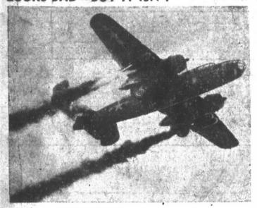
Nó, this B-25 medium bomber, the type now being used at Pampa army air field, is not on fire. The flames and smoke streaming from it are from rocket take-off units, used to assist heavily-laden planes into the air from short runways. Photo was taken at Wright field, Dayton, O., where the AAF materiel command made successful tests of
