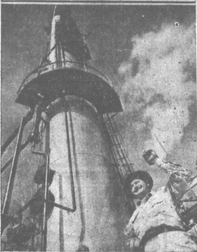
MILLIONS MORE GALLONS of 100-octane aviation gasoline for Uncle Sam's super bombers blasting Japan's war industries will flow from this huge plant recently completed by The Texas Company on the Pacific Coast. This rounds out a nationwide program of refinery expansion by Texaco to meet vast wartime demands. Officials say the new plant is also capable of producing new super aviation fuels, even more powerful than 100-octane, as soon as the armed forces give the go-ahead signal. Photo shows part of giant super fractionator tower.
