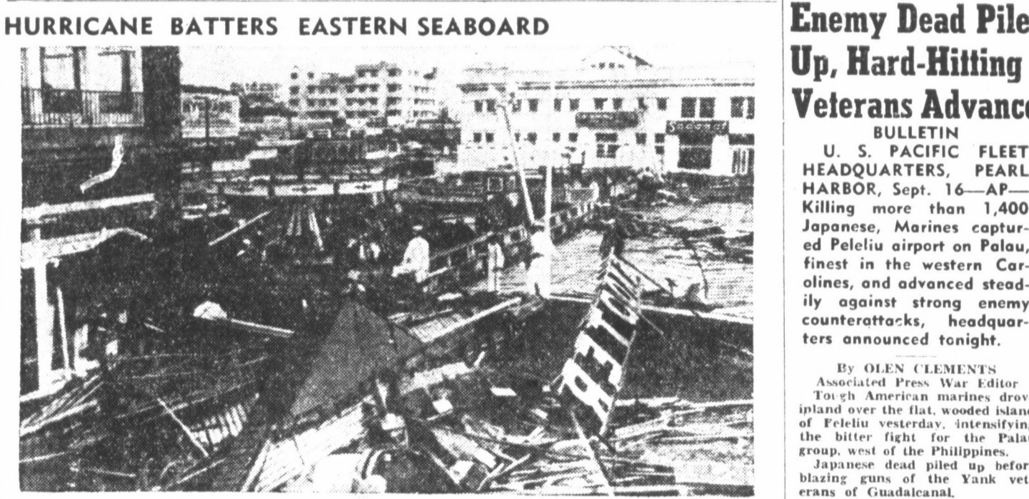
Typical of the devastation wrought by the hurricane which battered the eastern seaboard, taking $30,000,000 damage and a score of lives, is this waterfront view of Asbury Park, 35 miles south of New York. A carousel stands in the midst of the debris. Atlantic City, 60 miles to the south, was also badly hit. (NEA Telephoto).
