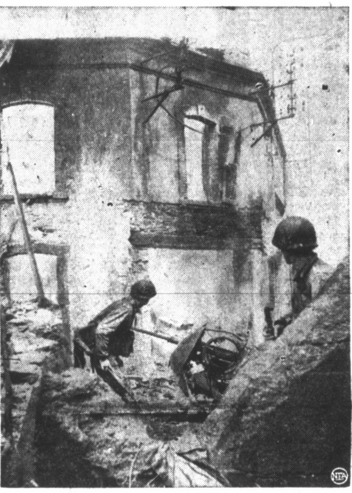
Combat engineers move in on an objective somewhere in Normandy, still under fire of German artillery. They take cover in ruins of buildings already hit.
