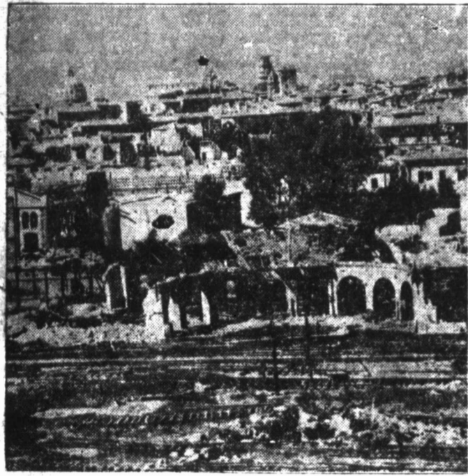
Above the battle-scarred city of Pisa, the famous Leaning Tower, in the center background, stands untouched by attacking planes. Wreckage of railway yards, target of Allied raids, are shown in the foreground of the photograph made by the U. S. Signal corps. (Released by War Department.)
