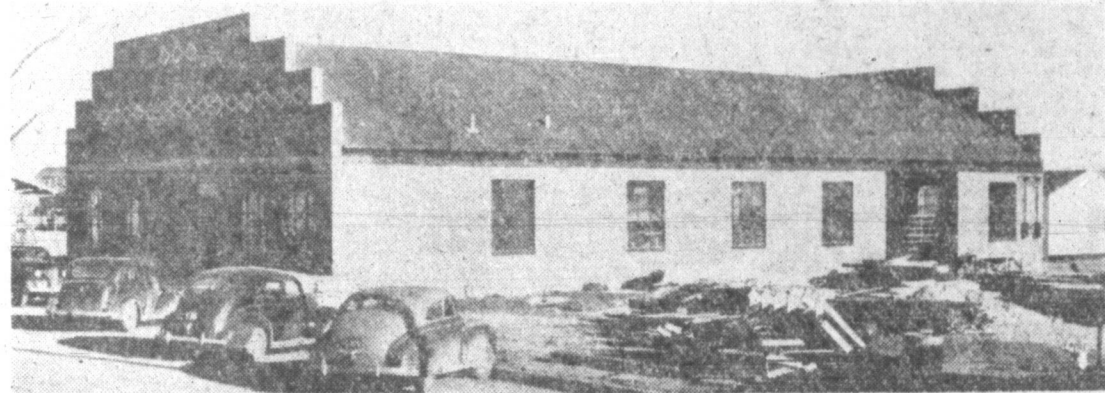
Burnett's Cabinet Shop (pictured above) is completely equipped and staffed to build and install wood and steel truck beds in three days. Materials used are of the best quality. The work is priced economically. The shop is located at 311 East Tyng. (Photo by Smith Studio).
